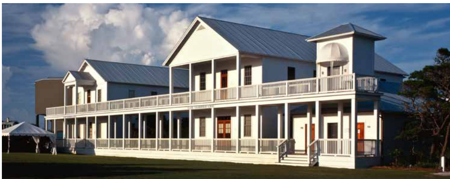
The Seaside Neighborhood School illustrates how a school can be integrated into a neighborhood and use less land than a typical school. Photo courtesy Seaside archives
